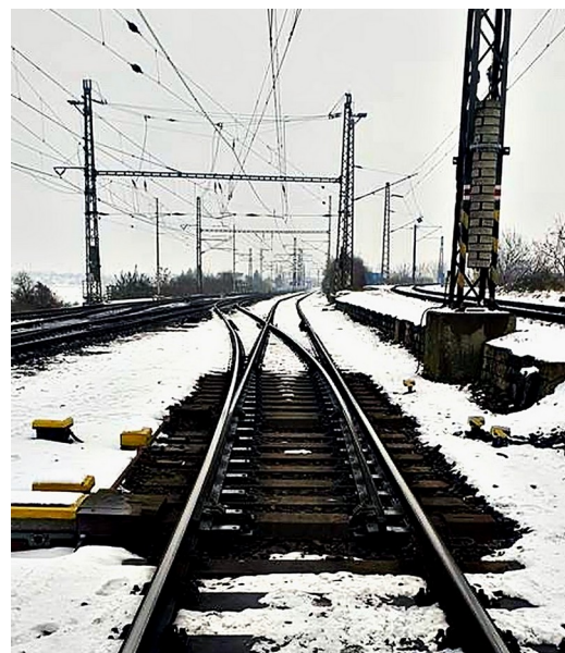
Turnout with MAGUS EOv – view along the track
